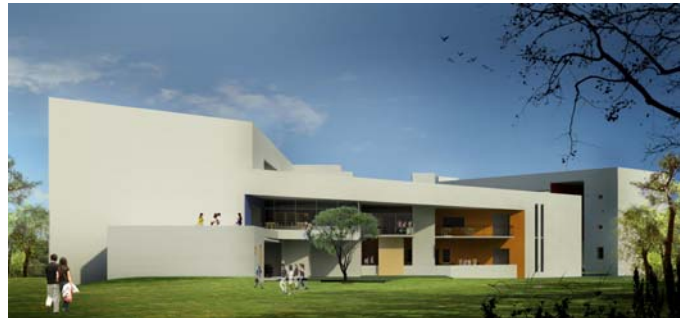
SCHOOL OF STUDY BUILDING
